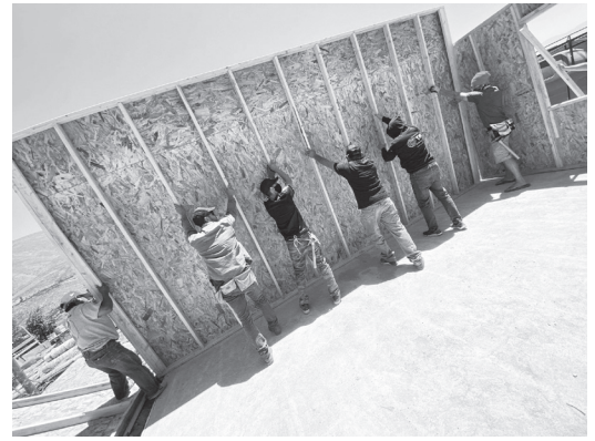
Putting up the walls.
