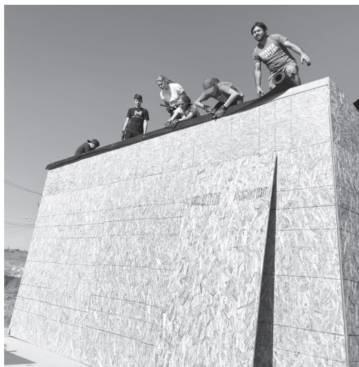
Working on the roof.
