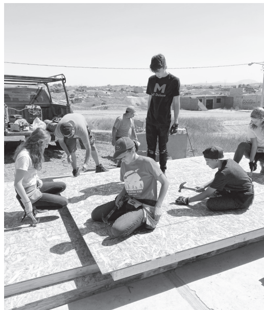
Putting together the walls
